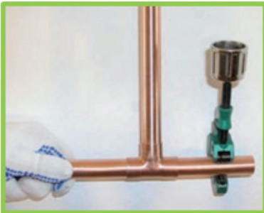
Cutting tube: Use only a wheel cutter.
